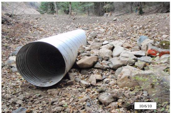
**Photo 3b.** Cecilville/Taylor Road #1, site #42, similar view as above, after implementation. The channel has been excavated with 2:1 side slopes below the crossing, and a 36 in. diameter  $\times$  40 ft long culvert installed. Rock armor has been placed along the outboard fill for fillslope protection.
