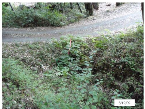
**Photo 11a.** Butler Flat, site #102, before implementation. View from TOP of the crossing, looking downstream towards the inlet of this undersized and nearly plugged culvert.
