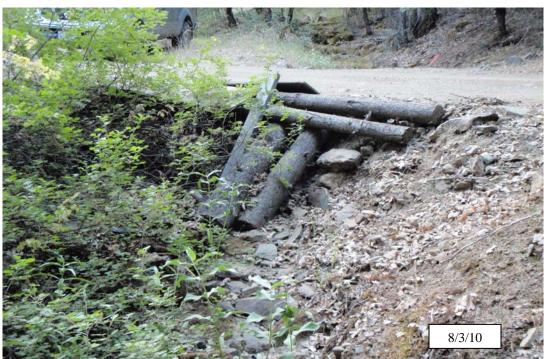
**Photo 3a.** Cecilville/Taylor Road #1, site #42, before implementation. View from the bottom of the site, looking upstream at a crossing of a Class III stream. Prior to treatment, there were two, mostly plugged culverts at this site and a plywood/debris supported outboard fillslope.
