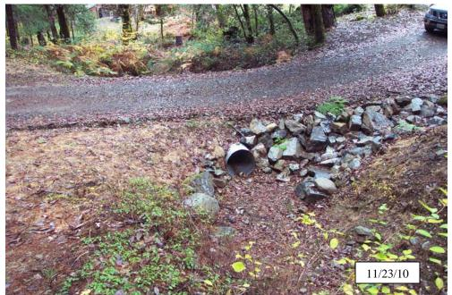
**Photo 11a.** Butler Flat, site #102, similar view as above, after implementation. View from TOP of the crossing, looking downstream at the new culvert inlet. The channel has been excavated with 2:1 side slopes above the crossing, and a 24 in. diameter  $\times$  30 ft long culvert installed. Rock armor has been placed along the right approach, lead-in inboard ditch to minimize future scour from an active spring.
