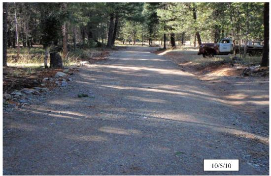
**Photo 4b.** Finley Camp Road #1, similar view as above, after implementation. The road has been widened and road rock was applied. The inboard ditch (on right) was widened, deepened and armored in order to effectively convey ditch/stream flow through the site.
